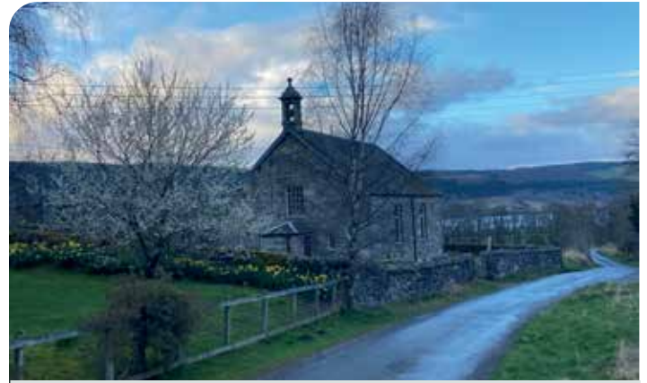
The converted church which is now being kept warm by a Grant heating system
