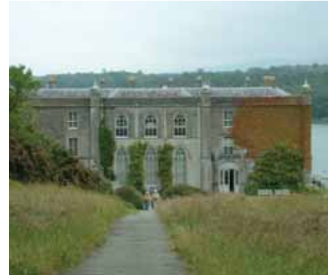
Plas Newydd is swapping oil boilers for a marine source heat pump
