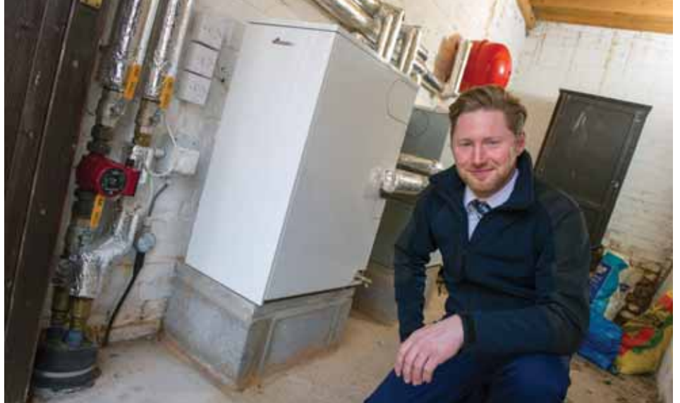
Daniel working on the award winning installation
