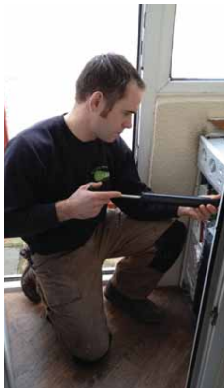
Flue gas analysis – a smoke pump has a very definite place for years to come says OFTEC inspector Norman Armstrong
