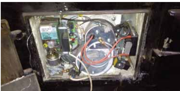
“A burner ready for service – four nuts and the head is out – it’s a 20-minute job – nozzle change, fan clean and new filter – no wicks or clogged up bundy tube,” says Barry
