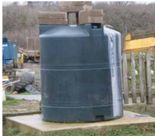
Tanks need attention – this much overburdened one in Devon (perhaps an attempt to stop it floating away in the recent floods) ... has evidence of a white chalk like appearance
