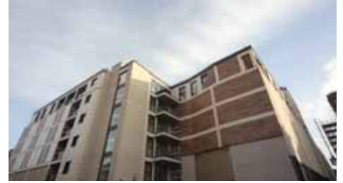
Ecodan heat pump technology is being used at Kingston Heights to produce zero carbon emissions
