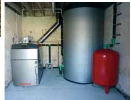
The new boiler room – complete with a SolarFocus 60kW log boiler
