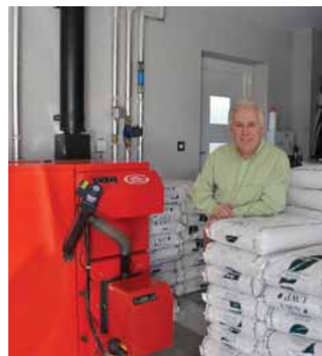
Eco-friendly property developer Colin Goodwin with his new Grant Spira wood pellet boiler
