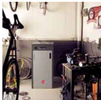
A biomass boiler is normally installed in a garage or utility room where it is connected to a wet radiator system
