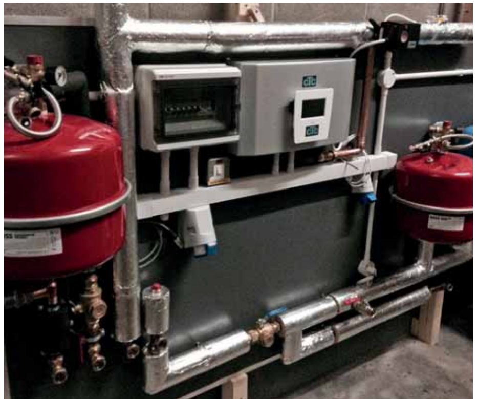
The Spire Renewables heat pump kit includes a pre-plumbed, pre-wired backboard
