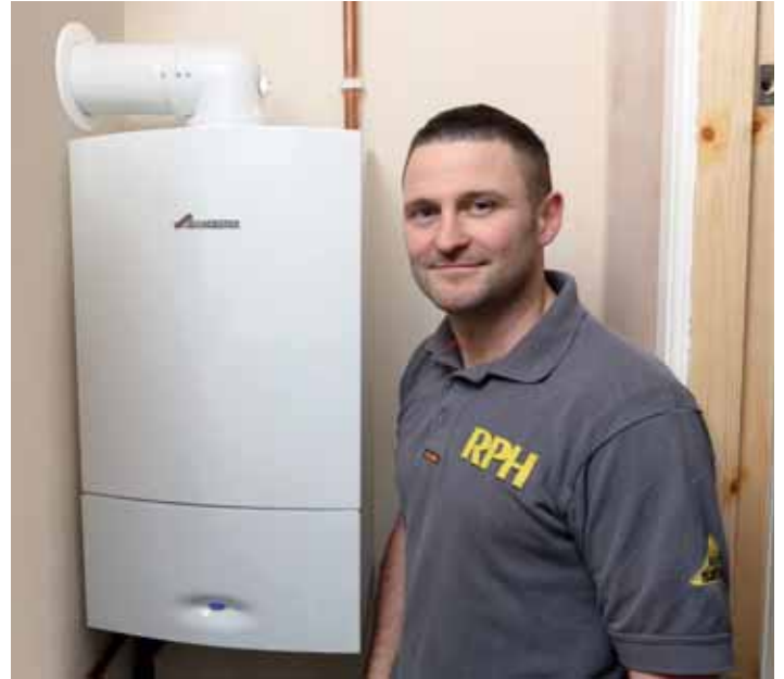
The installer cash-back incentive applies to Worcester products installed by the end of 2015
