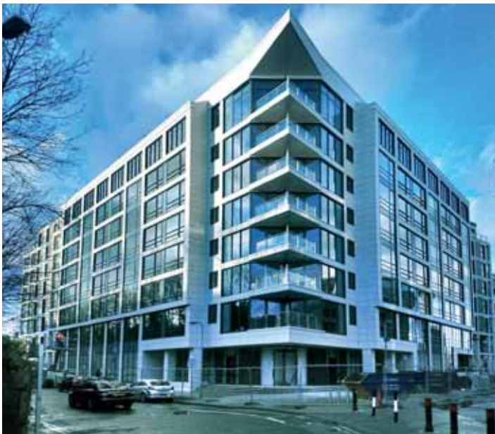
The £70 million Kingston Heights development which now gets its renewable heating and hot water from the River Thames
