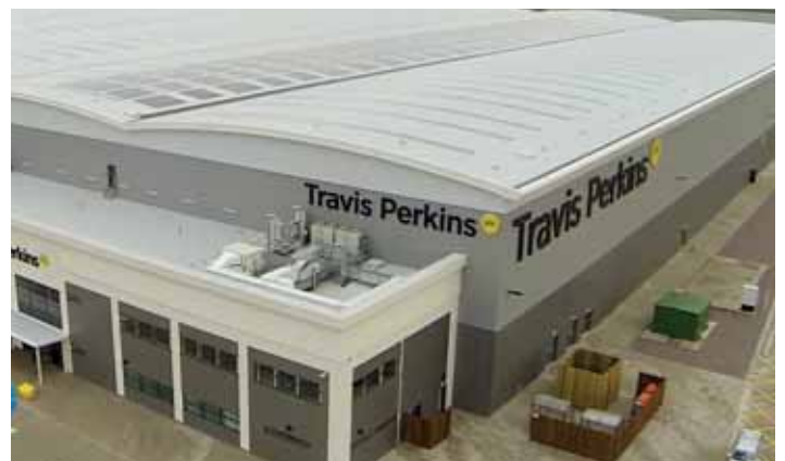
Solar panels fitted by Solarlec at Travis Perkins' regional distribution centre in Appleton, near Warrington, Cheshire.
