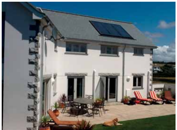
The Viessmann solar system comprises three solar panels on the south facing roof, working in tandem with the oil boiler
