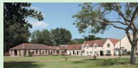
Equipped with an environmentally friendly solution capable of providing heating and hot water to the whole site including farmhouse, visitor centre, function and event rooms, offices and a flat
