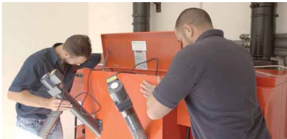
Installer Scott Lemon fits the biomass system's hopper
