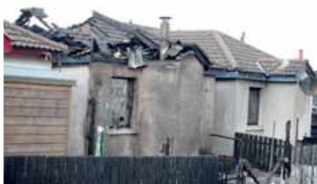
The bungalow in Belvoir, Belfast, destroyed by an oil tank fire
