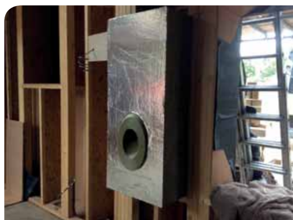
The Ignis Protect being installed
