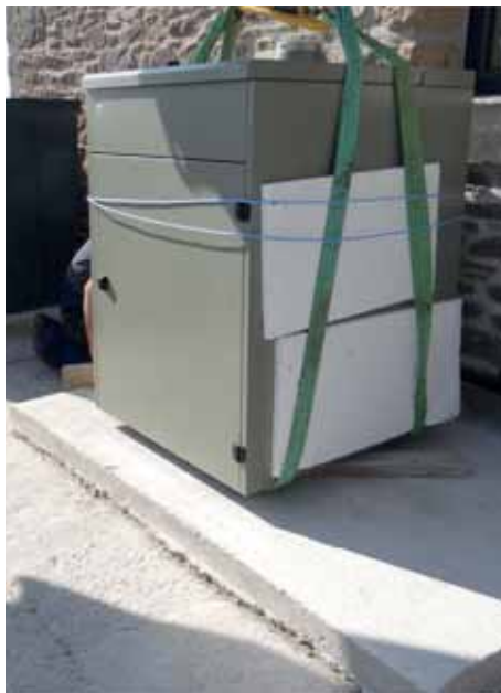
Step 2: The Vecta boiler is craned into position
