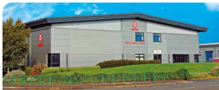
ABGO's new UK distribution centre and headquarters
