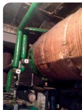
One of the most challenging oil heating jobs which Maxiflow has encountered recently was to strip out and replace a 60+ year-old oil boiler – insulated with a complete covering of asbestos (pictured above) – in a 15th century country mansion. With the company's all-round construction and heating expertise, Maxiflow treated it as a routine assignment...
