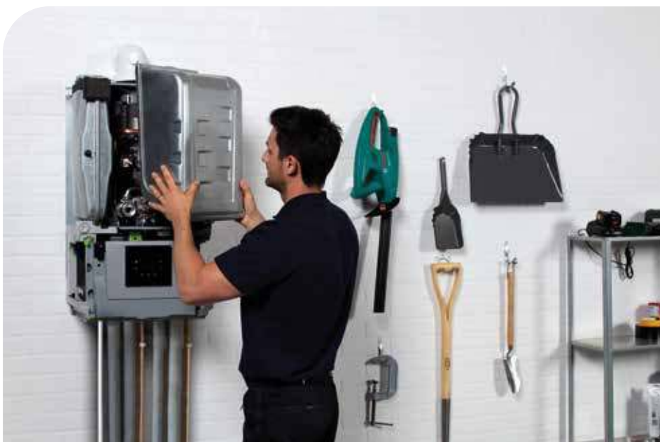
Lockdown has limited boiler checks
