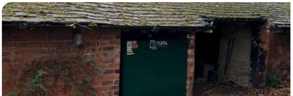
Tuffa designed and built a steel bunded fire-protected tank to fit into an existing store to meet a customer's exact requirements
