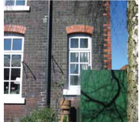
A flue terminal protruding from an appliance must be located at least 1.8 metres from an oil storage tank
