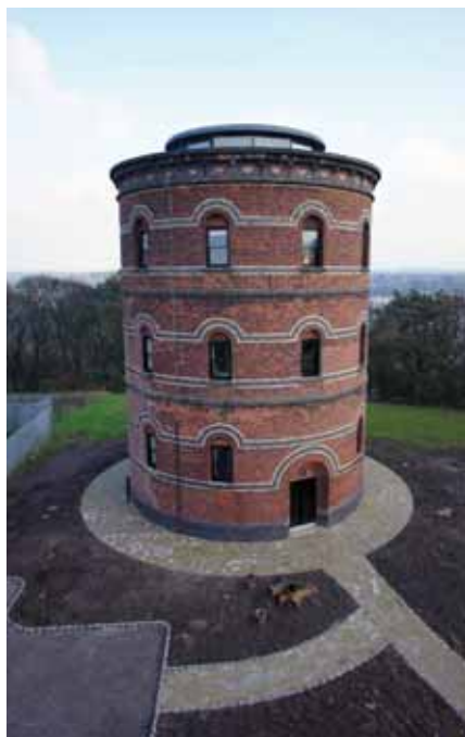
The conversion of the water tower was featured on Channel 4's Restoration Man earlier this year
