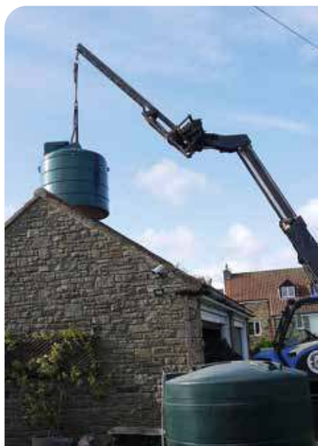
Lifting the new tank into place
