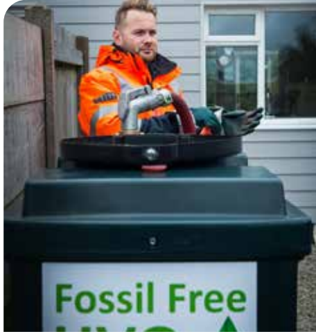
On site in Cornwall at an HVO trial set up by Mitchell and Webber
