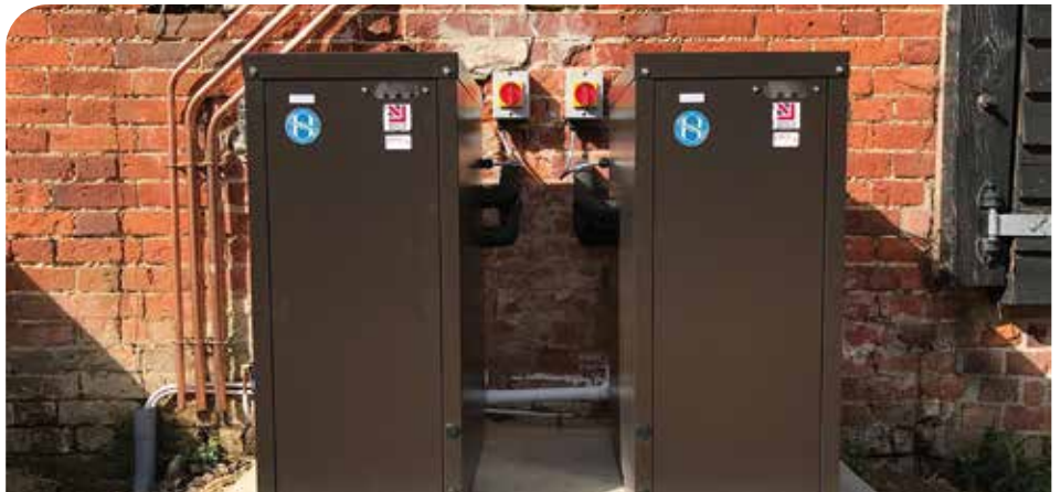
Hounsfield's oil-fired boilers
