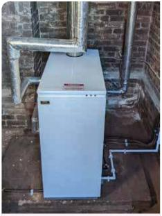
Firebird's Envirogreen C100 condensing boiler
